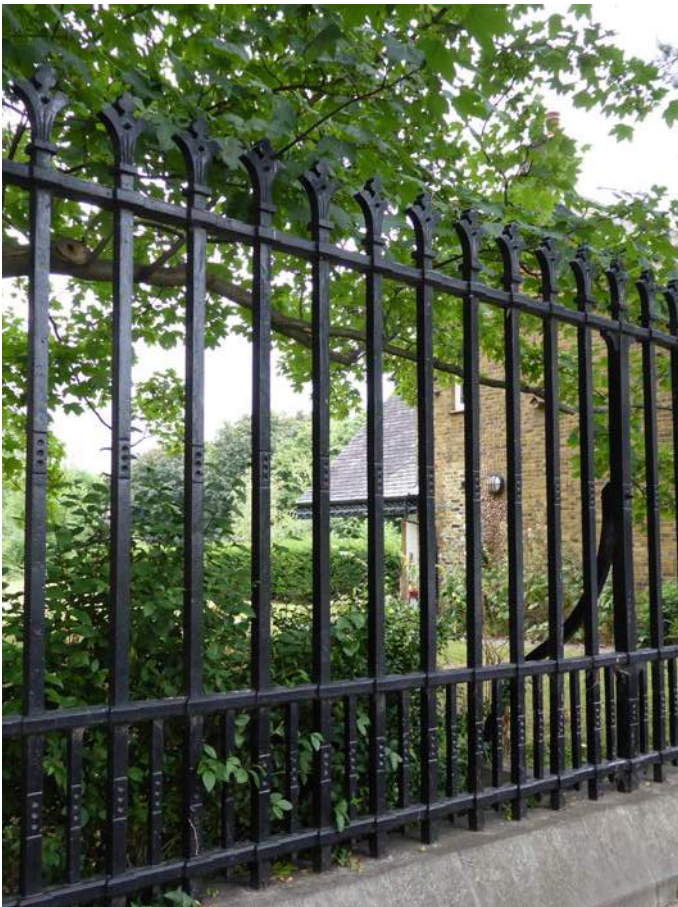
Railings to The Lodge
