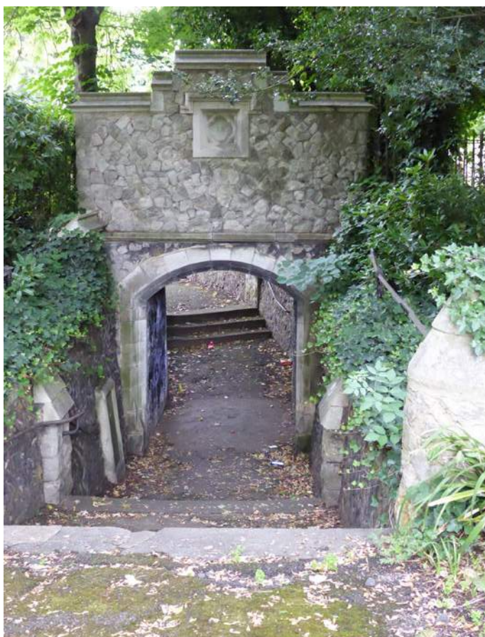
The tunnel beneath Church Path
