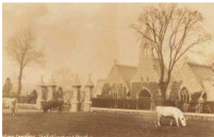
Victorian view of original entrance, courtesy of Bruce Castle Museum, Haringey Libraries, Archives and Museums Service
