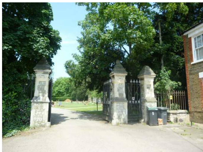
Entrance gates and gatepiers, Cemetery Road
